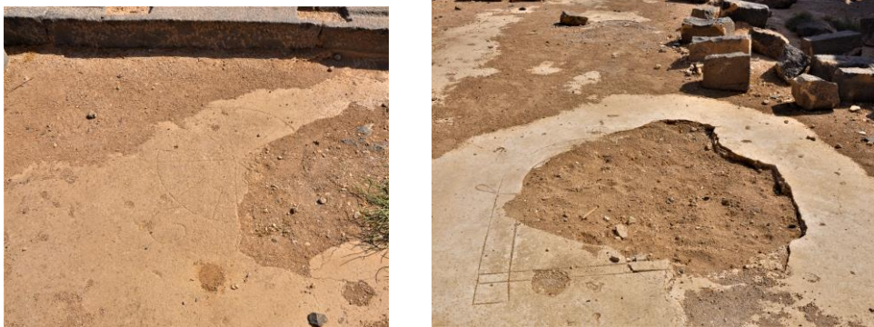
Figure 45: Floor of West church. Shows the plaster layer that would have been prepared as an underlayment for a mosaic floor. Author
