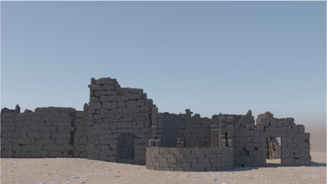
Figure 49: 3D perspective presents the ant eye of this church, it shows the apse and doorways, also the corbeling construction method. Sources: by Author.
