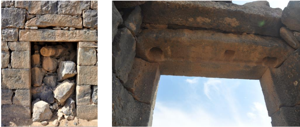
Figure 42: Southwest doors details; door's hinge and lintel inscription(cross). By Author.
